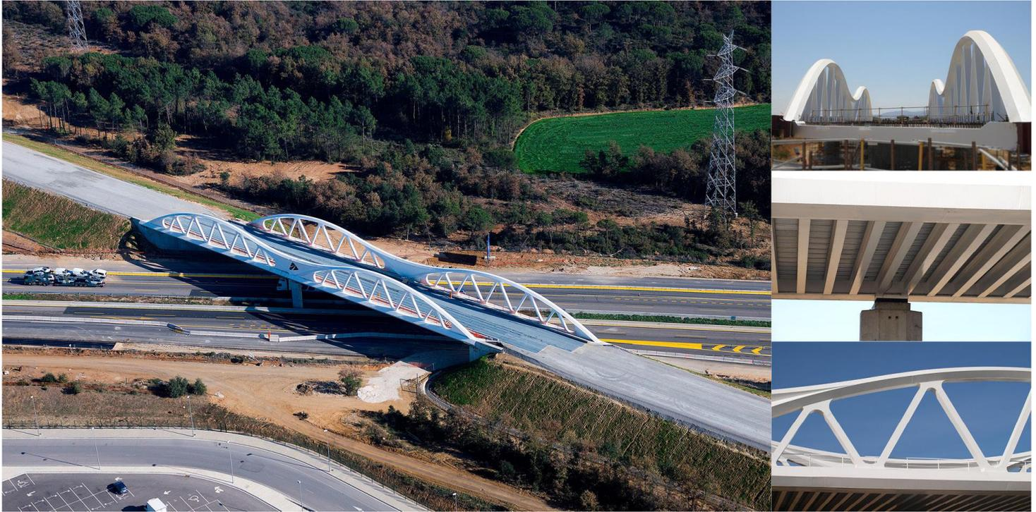
The structure consists of a single two span deck of 53.0m + 53.0m between axes giving a total length of 106.0m. The structure has a marked skew and therefore the axis supports on the piers and abutments offer an angle of 34.3° on the high speed train line. The width of the deck is a constant 15.70m.
